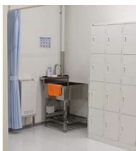
Handwashing sink, air dryer
